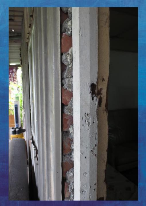
Metal sheets weather-proof sub-standard brick and mortar walls
