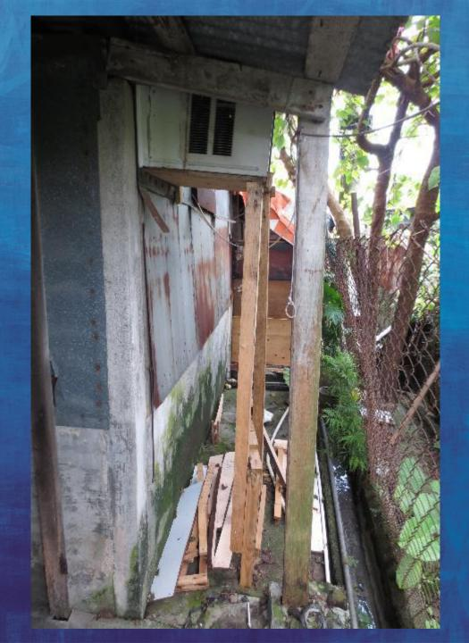
The rotting roof is held up by beams propped on the wet floor.
